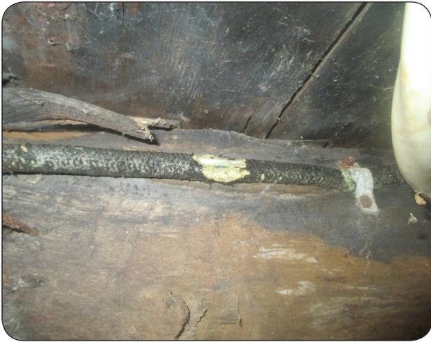
**Figure 5.** Rodent damage on electrical cable.
