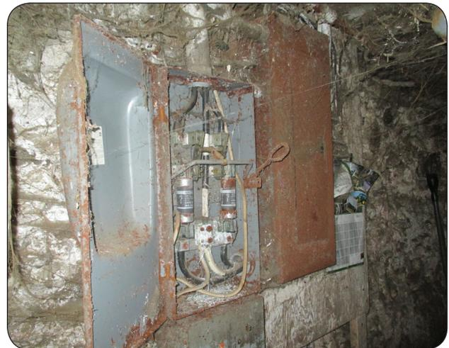
**Figure 4.** Corroded disconnect panel.
