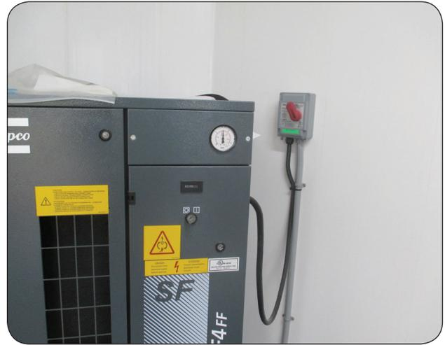
**Figure 8.** Hard-wired compressor.
