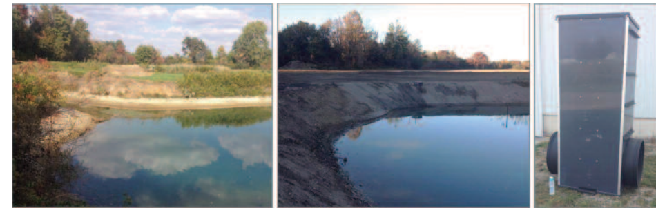
West irrigation pond outlet before (left) and after (center) and an 8' in-line water control structure (right) was installed to utilize a bottom draw mechanism to reduce the water temperature leaving the pond and entering the wetland downstream.
