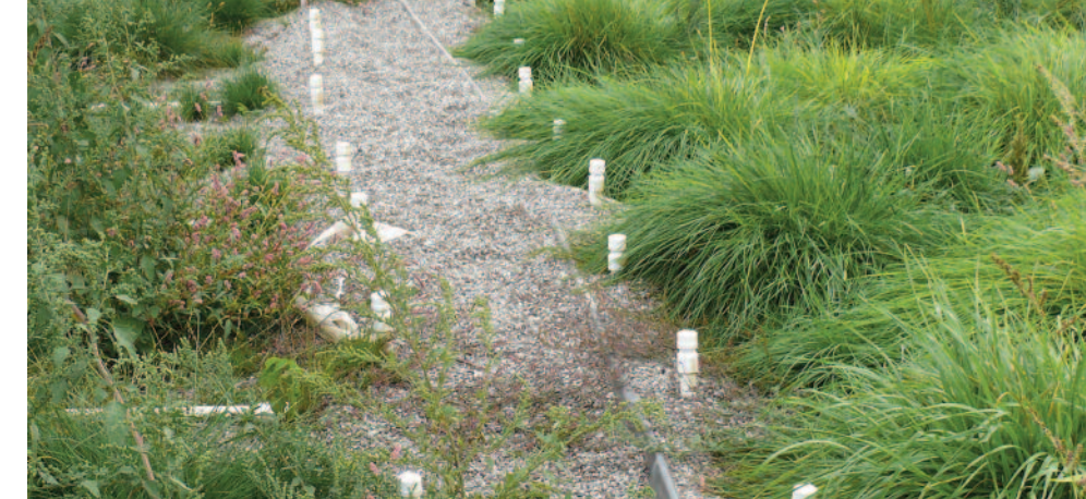
This vertical wetland successfully removes pathogens from greenhouse effluent.
