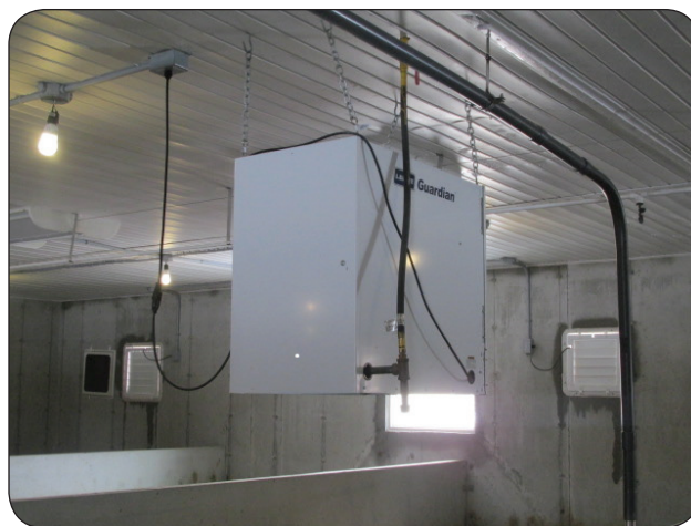
Figure 8. Radiant tube heater suspended in barn.
