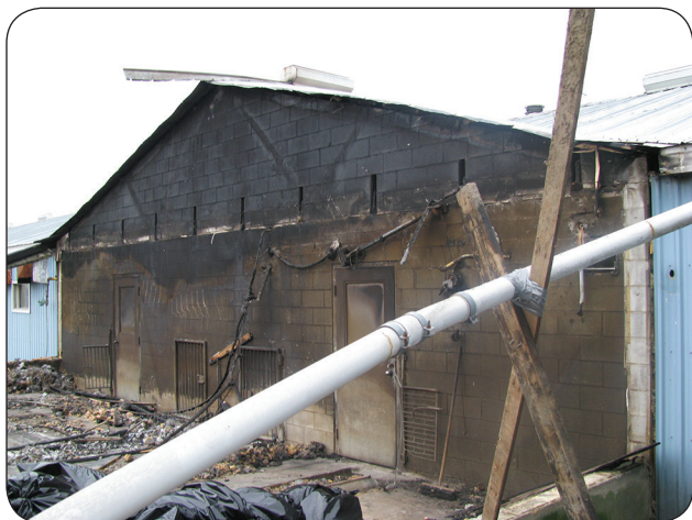
Figure 7. Example of an intact firewall that did its job and prevented fire from spreading through the barn. Source: R. Drysdale, Farm Mutual Reinsurance Plan.
