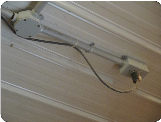
Figure 2. Temporary electrical equipment plugged into receptacle in livestock area. Source: Heartland Farm Mutual, Ontario.
