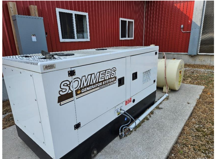
Photo of GenerLink transfer switch and standby unit on a dairy farm from Sommers Generators
